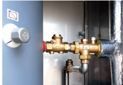
Mischventil Mixing Valve
