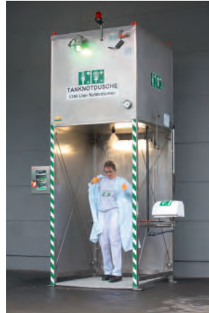
Tanknotduschen Tank safety showers
